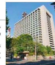
Central Gov't Bldg. No.2
