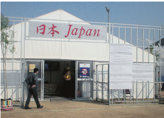
Photo 3 Japan Pavilion in Ubuntu Village.
