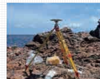
Construction of a 2nd order triangulation point (Hirase Island, Kagoshima Pref.)
